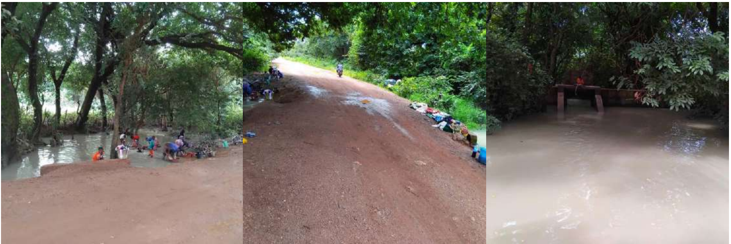
Photograph 10. Fandjia stream at Damissakoura (no bridge and stream-closing valve)
