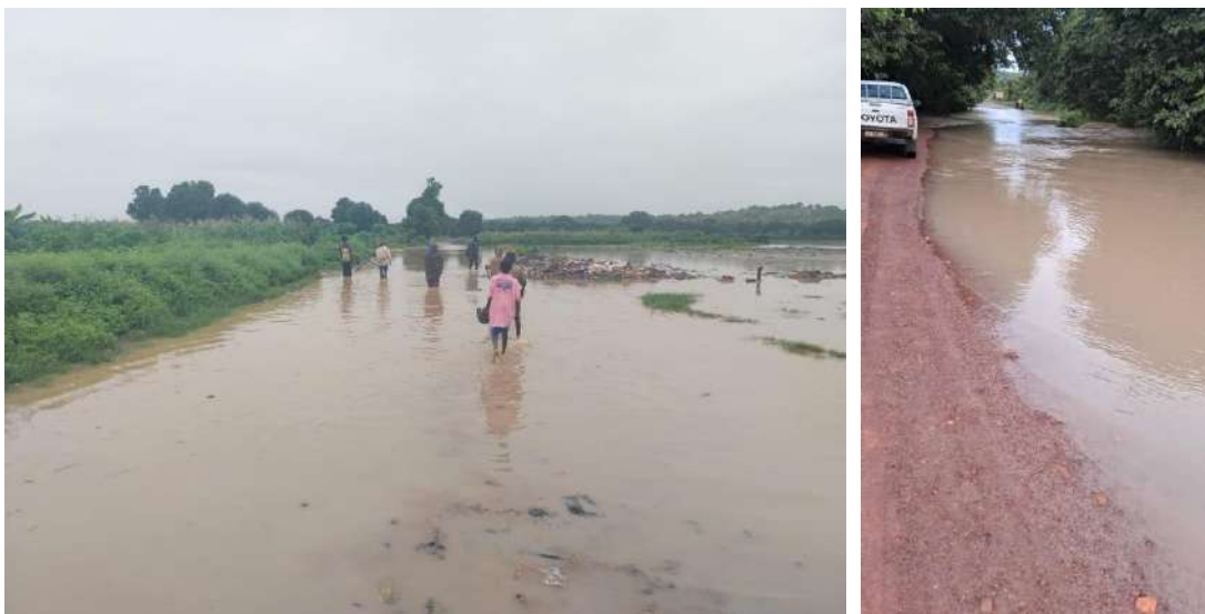
Photograph 11 : Illustrations of the flood zone on the RN 32 during the rainy season field mission
