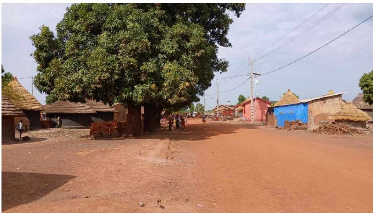
Photograph 54: RN 32 at Nounkounkan and power lines under construction at the time of the study, Source: Insuco, April 2025
