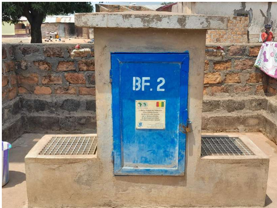
Photograph 53 : Drilling station at Balato, Source: Insuco, 2025
