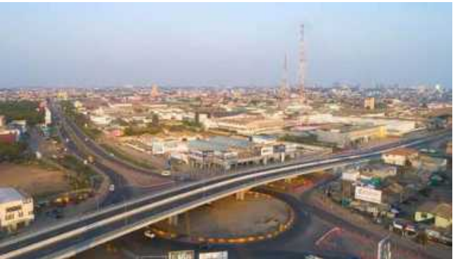
Project under construction Phase 2: Construction of a north-south flyover; upgrading of the existing Obetsebi Lamptey roundabout to ground level; and implementation of adjacent drainage works.
