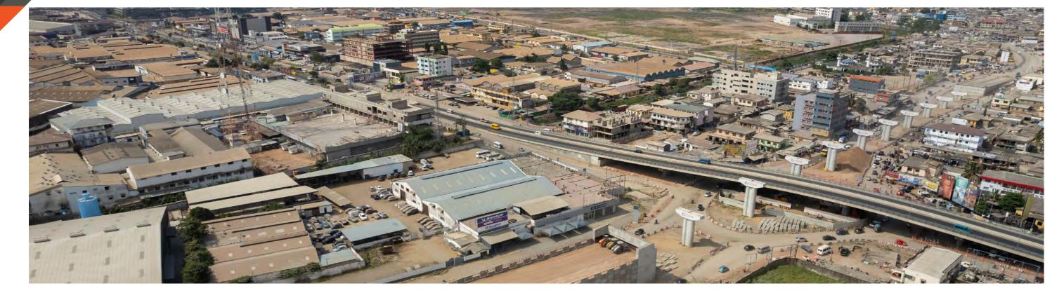
> Phase A includes the upgrading and widening of the roundabout and its approaches, as well as the construction of an east-west viaduct of approximately 390 metres in length that will connect Winneba Road (Dr. Busia Highway) and Graphic Road. This phase will also include drainage improvements to reduce the impact of frequent flooding in the area.
