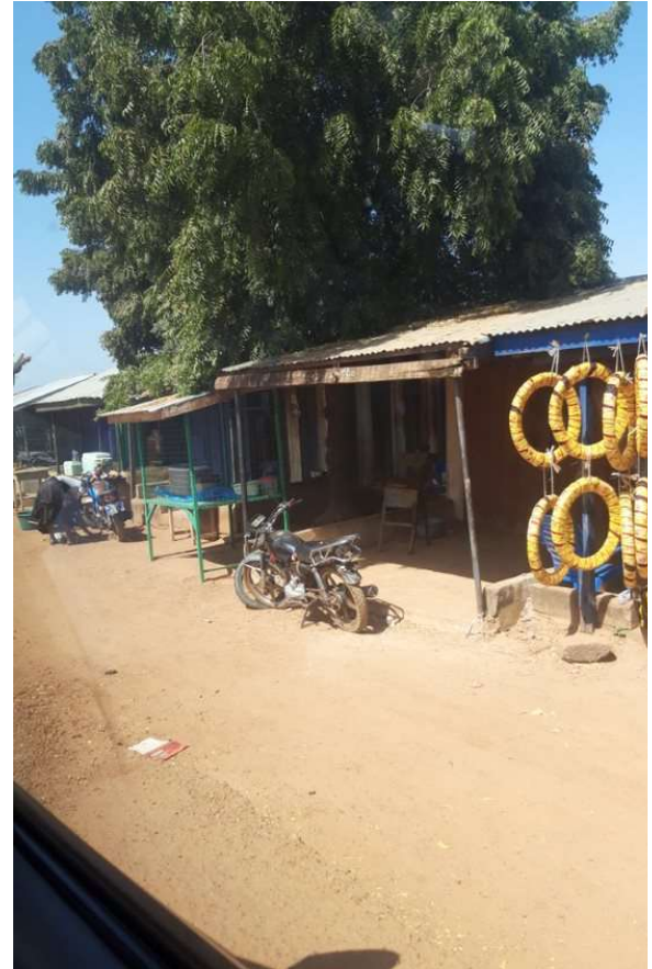
Second example of metal container temporary structure
