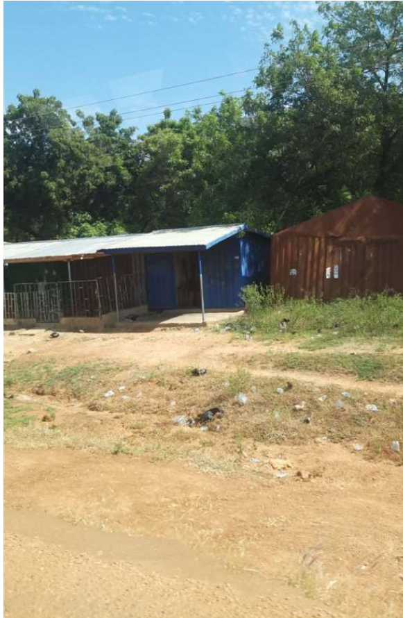
Example of metal container temporary structures adjacent to the road on outskirts of Bawku
